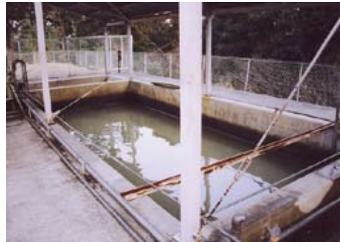
Oil-water separator. It purifies rainwater and wastewater and discharges them to the rivers.
